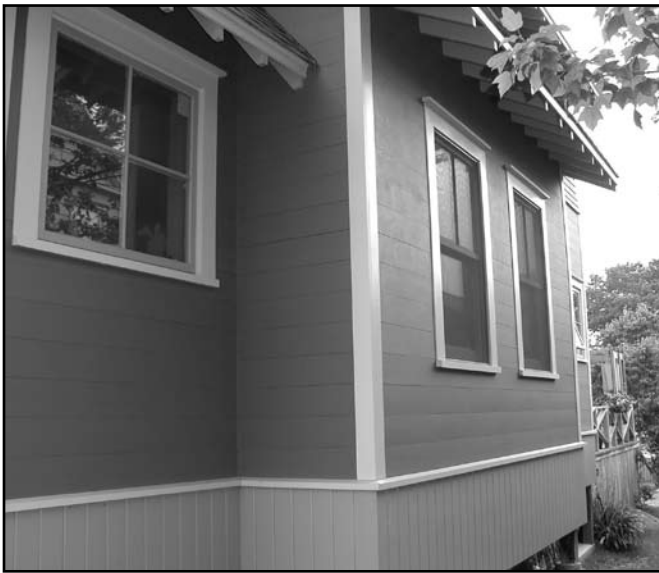
THE JOHNSON'S PEAKS ISLAND COTTAGE: WHITE PINE SIDING.
